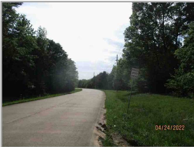
Street View Looking West on E.. 19th St.. Concrete Street.
