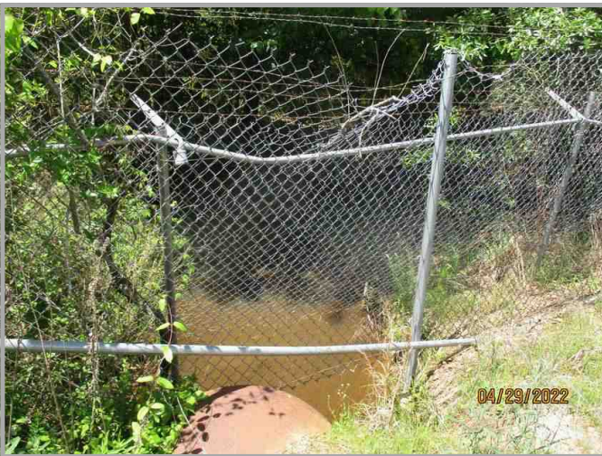
Drainage Ditch Crosses Tract approximately 3/4 toward the Rear of the Site.
