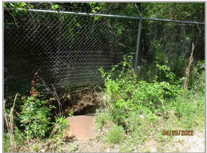
Drainage Ditch Crosses Tract approximately 1/4 from the Rear of Site.
